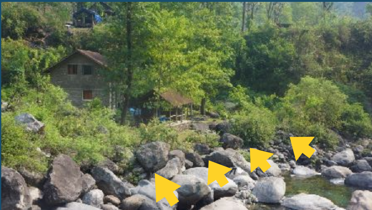
RIVER ENCROACHMENT TOWARDS ACPC BUILDING IN SISUWATAR. THIS RIVER ENCROACHMENT BECOMES MAJOR CHALLENGES FOR ACPC THAT NEEDS TO BE CONTROLLED QUICKLY
