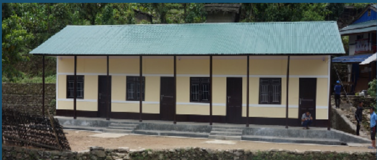
Completion of rebuilt of Shree Balkanya Adharbhut School in Hoyengla village
