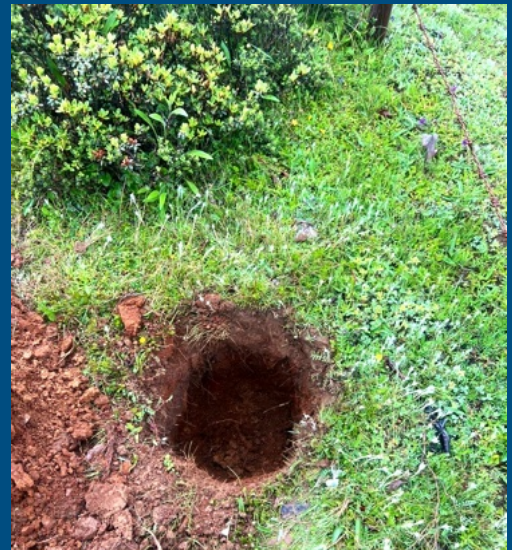
Pit digging one foot height and one foot length
